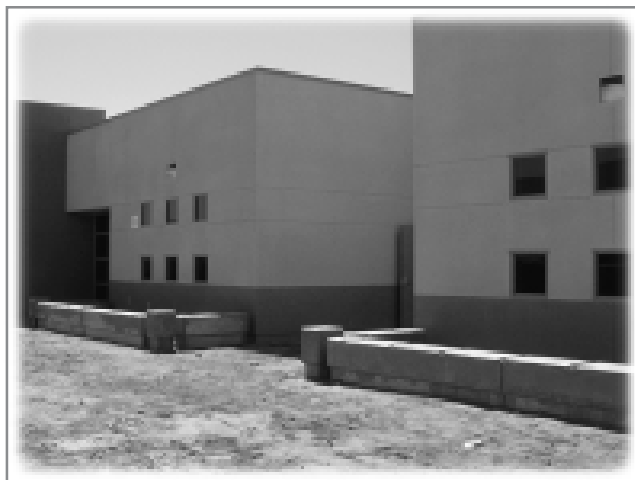
Buildings E & F
